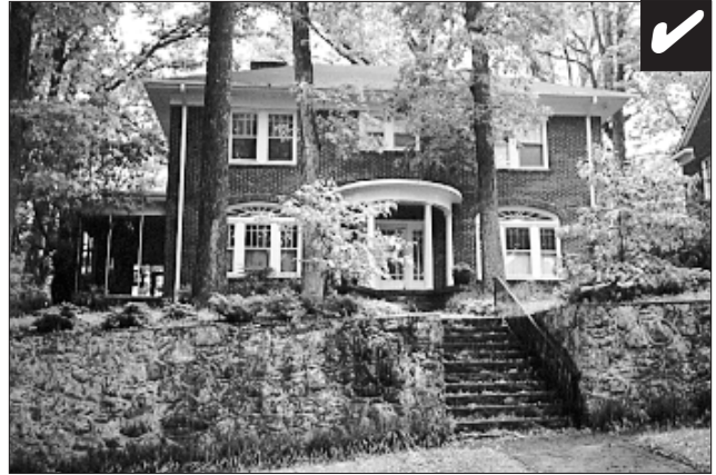
Masonry should appear similar to that used historically.
