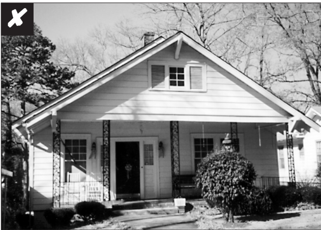
This porch has experienced an inappropriate alteration; wrought iron supports have replaced wood piers. Compare it with its "twin" in the photo below.
