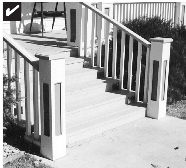
Where an architectural feature, such as this porch support and rail, is damaged it should be repaired rather than replaced. Compare this photo with the after condition at right where the porch supports have been remounted to the steps and a fresh coat of paint has been applied.
