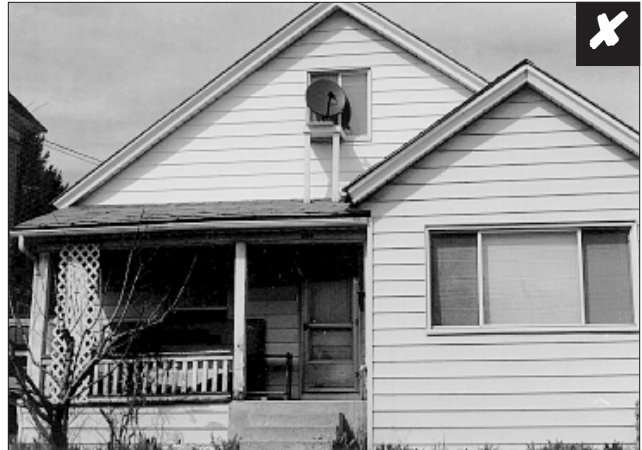
Maintain the historic ratio of solid-to-void on a primary facade. Significantly increasing the amount of glass on a character-defining facade, such as the window in the right of the photo, will negatively affect the integrity of the structure.
