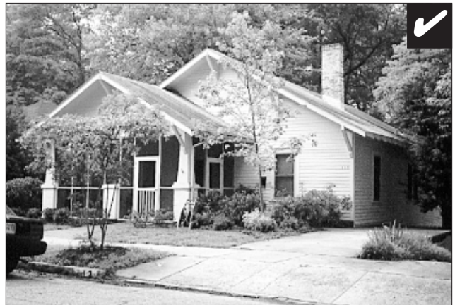
A new building should be visually compatible with historic structures.
