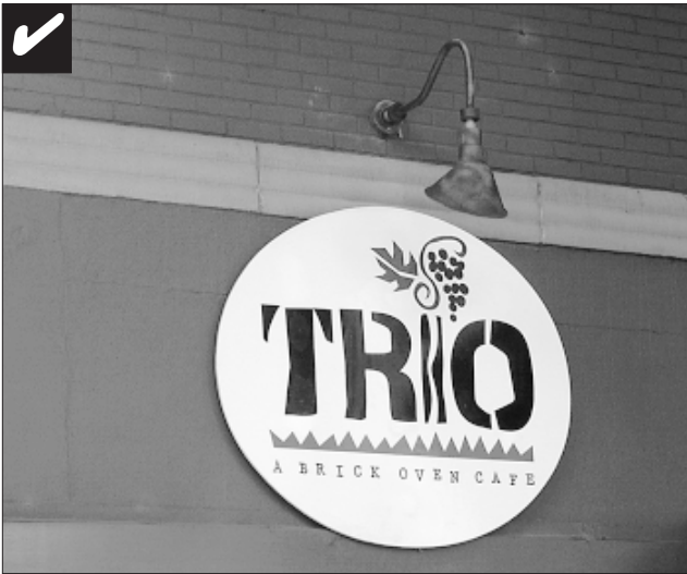
Lighting that is directed at a sign from an external, shielded lamp, is preferred.
