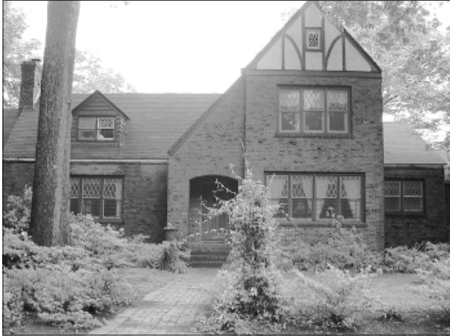
Masonry construction should be preserved in its original condition.
