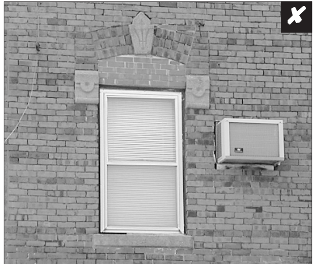
Do not locate window air conditioning units on a building's primary facade.
