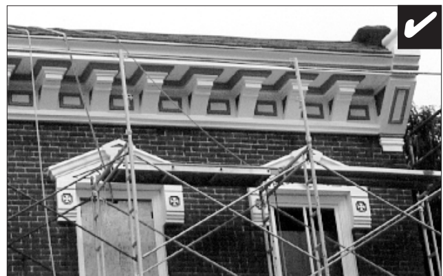
Repair only those features that are deteriorated. (Above photo is the "before" condition of the lower image.)
