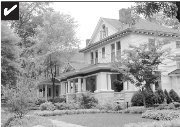
A new building should be visually compatible with historic structures.
