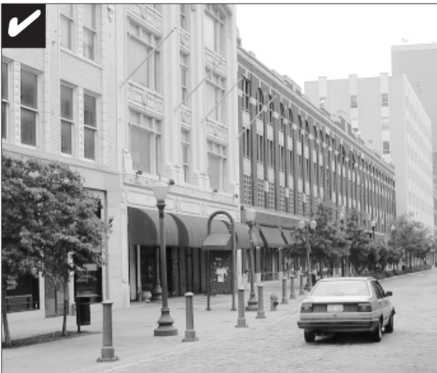
The overall building design of this parking structure is successful because it relates to the traditional buildings along the block in terms of mass, scale, alignment and materials.
