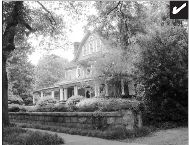
Maintain the historic height, form and detailing of a retaining wall.
