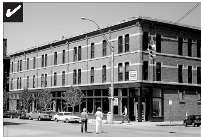
If a storefront is covered or obscured with a later alteration (top photo), then restore the storefront to its historic character.
