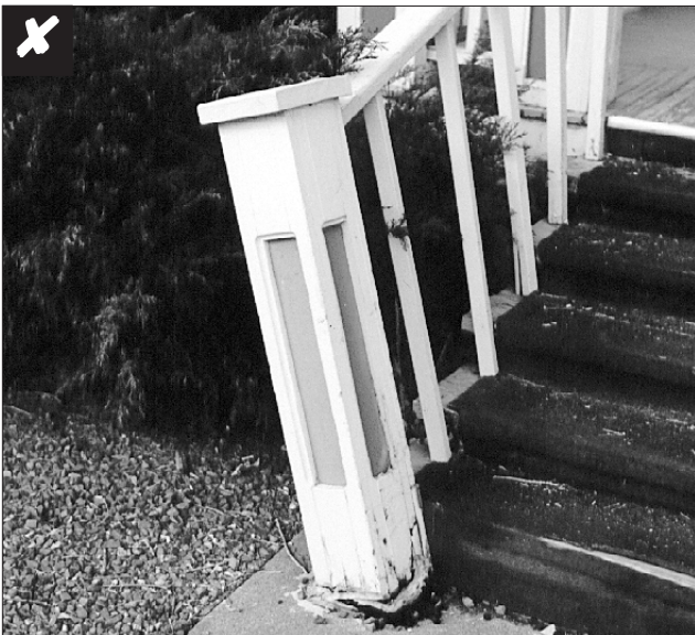
Where an architectural feature, such as this porch support and rail, is damaged it should be repaired rather than replaced. Compare this photo with the after condition at right where the porch supports have been remounted to the steps and a fresh coat of paint has been applied.
