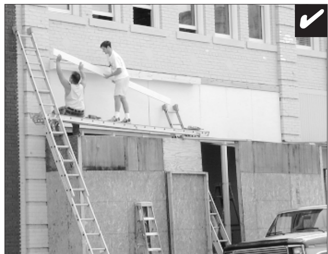
Replace missing original details in kind.
