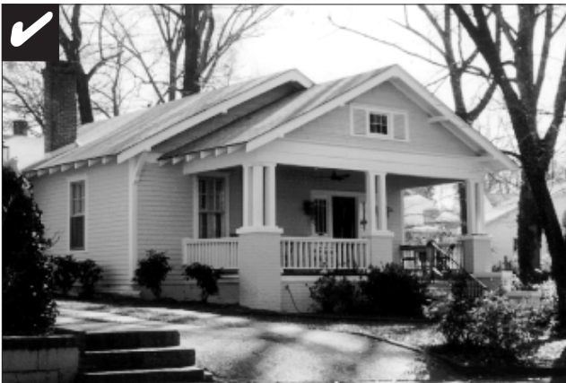
When replacing porch posts, use supports that are of adequate size. This porch reconstruction was based on neighboring houses of similar character and age.
