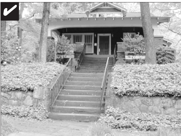
Preserve original retaining walls.
