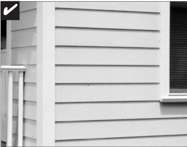
Newer, synthetic materials may be considered for a new structure, if they appear similar in character and detailing to traditional building materials.
