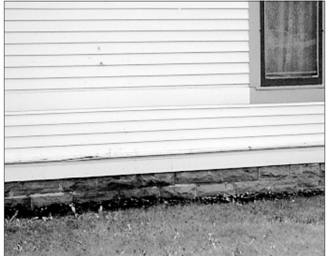
Make sure the soil or pavement next to the foundation wall slopes away and not toward the wall.
