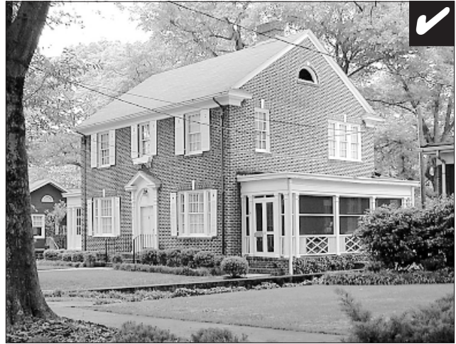
Preserve the original roof form.
