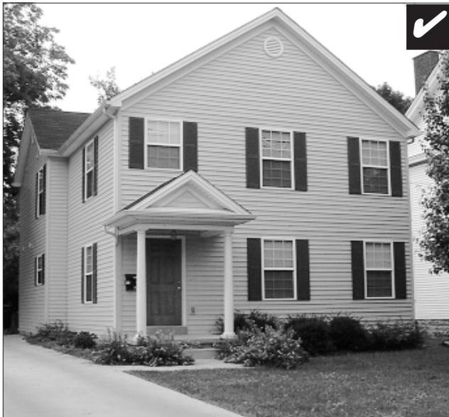
New construction should appear similar in mass and scale to nearby historic structures.
