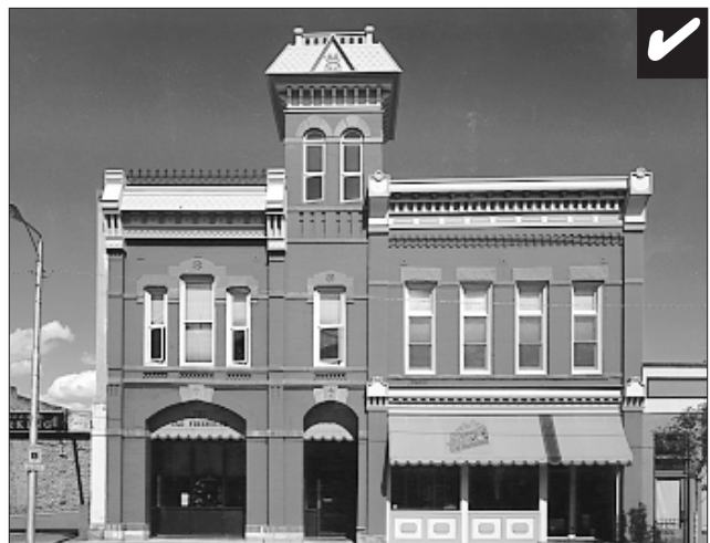
This rehabilitation preserves surviving details and reconstructs missing ones.
