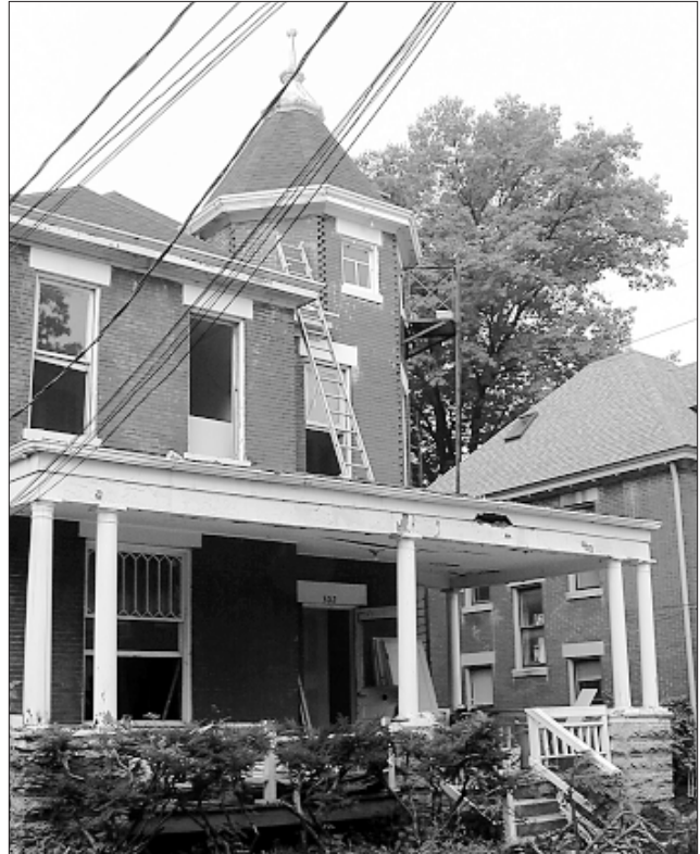
Repair deteriorated primary building materials by patching, piecing-in, consolidating or otherwise reinforcing the materials.
