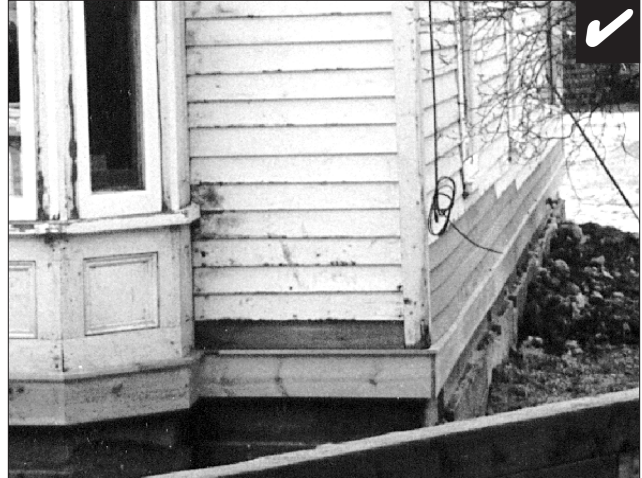
Repair wood features by patching or piecing-in new wood elements that match the original.
