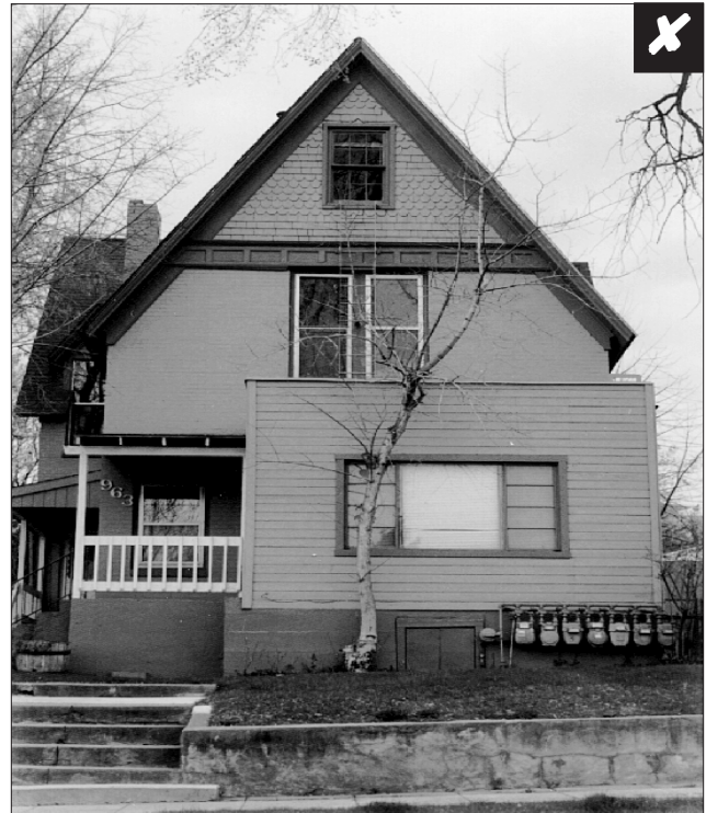
Design a new addition such that the original character can be clearly seen. This addition to the front of the historic structure is inappropriate.
