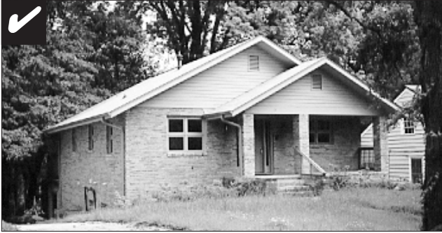
Masonry should appear similar to that used historically.
