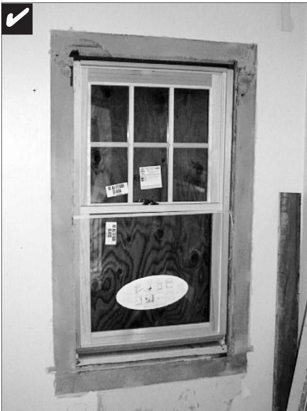
When window or door replacement is necessary, match the replacement to the original design as closely as possible.
